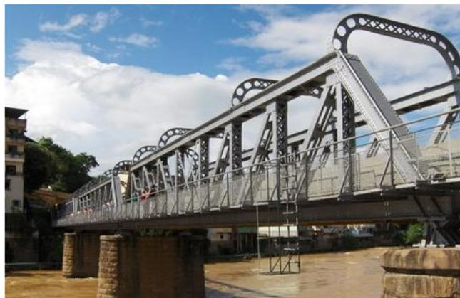
was manufactured in England in steps and sent to Brazil in various parts to be assembled here. There is a plate located in one of the columns of the structure of iron bridge that informs us:
